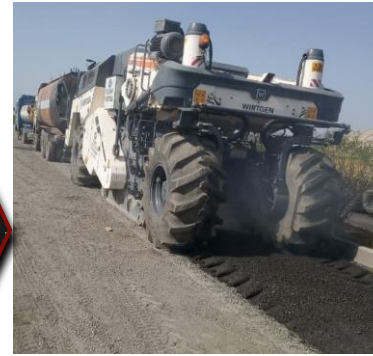
Milling & pulverisation by WR240 Wirtgen Recycler
