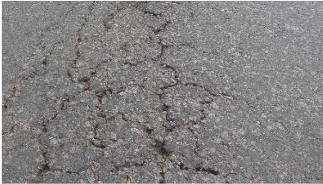
Alligator Cracks
