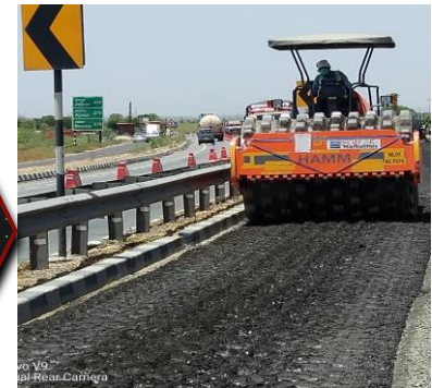
The sheep foot roller for compacting top layer
