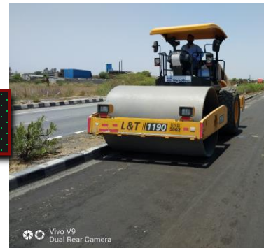
Compaction with Single Drum smooth wheeled soil compactor
