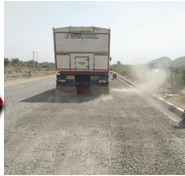
Spreading of Cement with Streu Master
