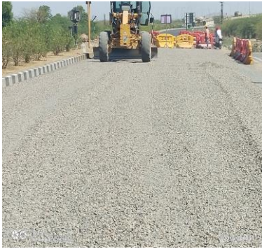
Spreading of Aggregate with Grader as per design proportion
